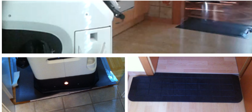
Fig. 2. Examples of ramps to overcome thresholds. Sometimes fixed with tape, which is certainly not wanted for permanent installations by users.
