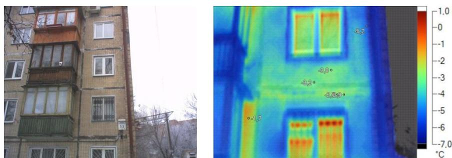
**Fig. 5** Photo and thermogram of characteristic zones of the enclosure constructions
