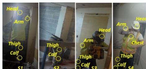
Figure 2. Subjects Working with Sensors (the sensors blocked are not circled)
