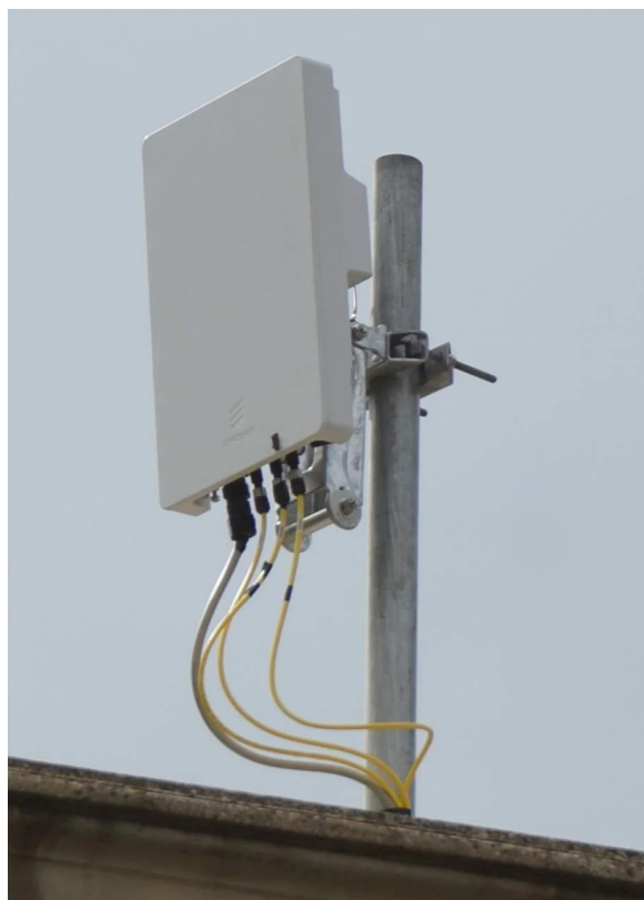
Figure 3: 5G antenna installed in Turin by Tim/Ericsson
