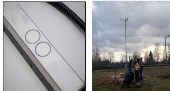
Figure 7: Ice/snow buildup sensor pilot model and its installation on testing ground.
