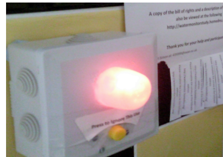
Figure 2: Our ambient-light installation
