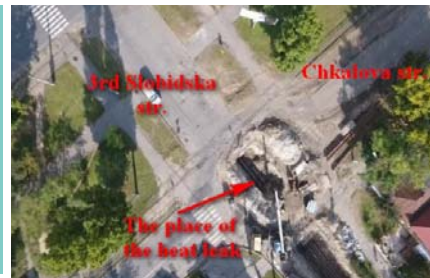
Fig. 12. The detected places of the local heat leak on the underground thermal pipe.
