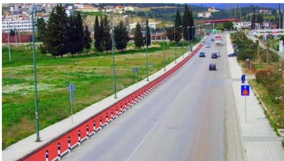
Figure 2: A view of a bicycle lane in the city of Lamia, Source: Dimos Lamieon [6].
