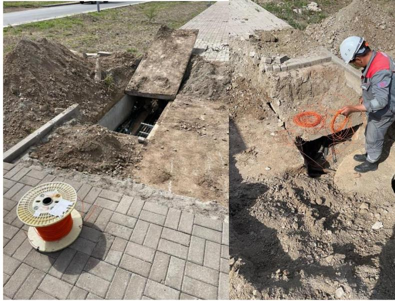
**Figure 7.** Installation of fiber-optic conductors
