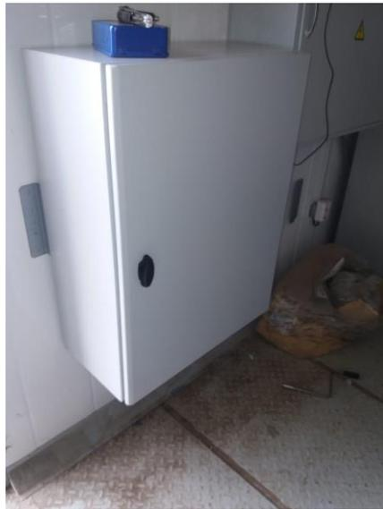
**Figure 5.** A universal wall cabinet with a processing unit placed inside a 10 kV DS room
