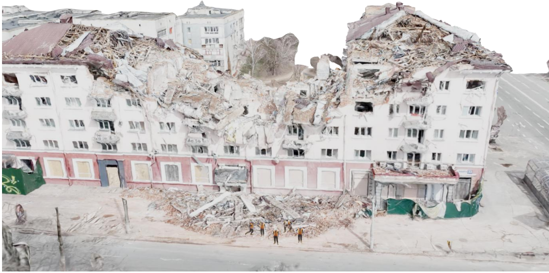
Figure 4: 3D model of a destroyed house
