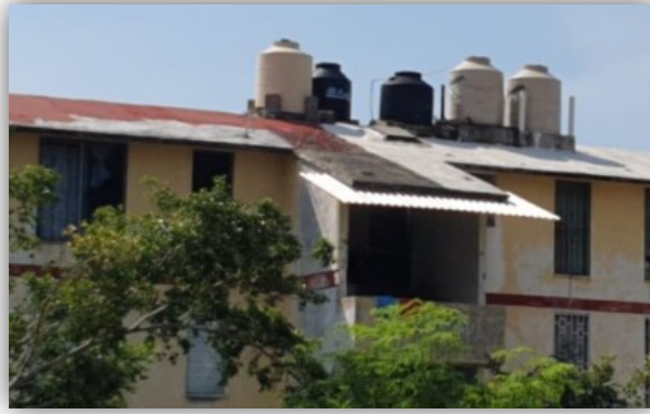
Figure 18: Location of water tanks in residential areas.
