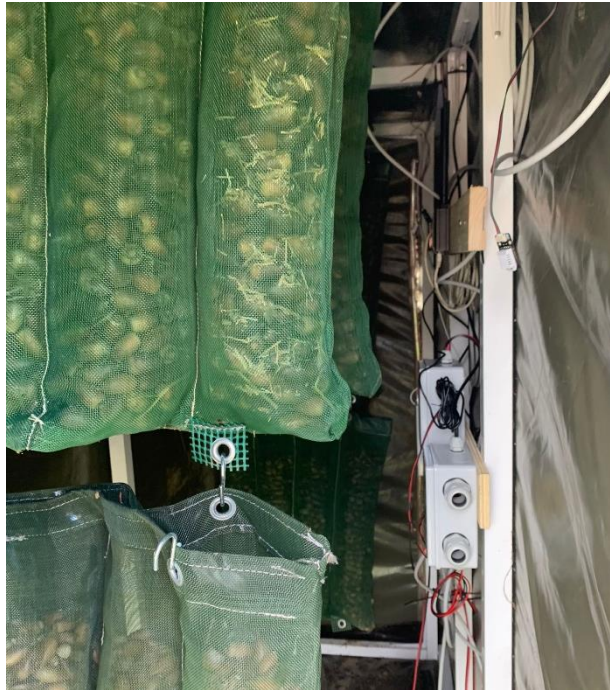
Figure 8: Boxes for processing the electronic signals.
