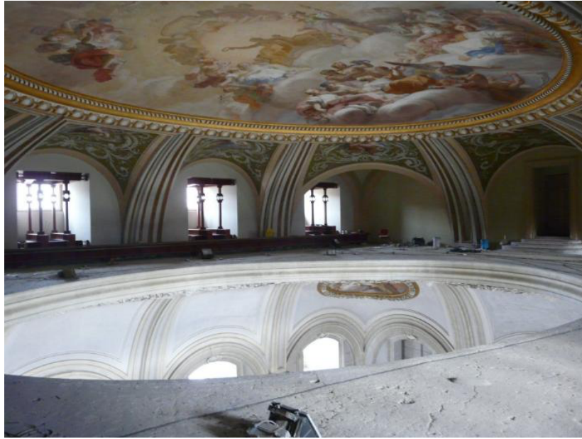
Figure 8: Double elliptical vault.
