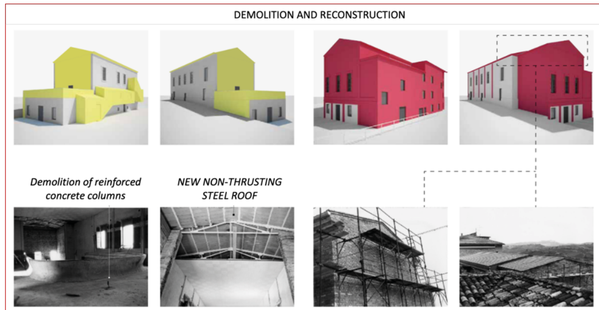
Figure 4: Structural constructive sequence: in yellow original design, in red final, actual, configuration
